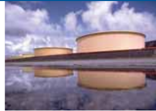
Waste Water Treatment
