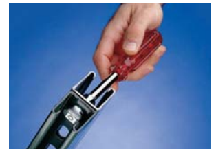
3. Tighten with 1/2" nut driver.
